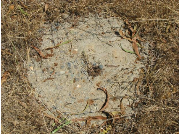
Concrete hole for metal pole on upper end
